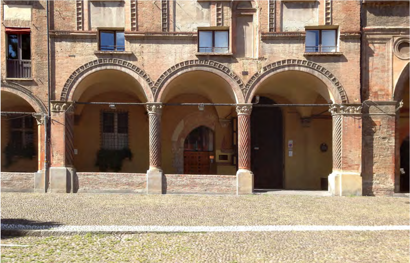
Fig. 16: Columns of the portico of Palazzo Beccadelli, Via Santo Stefano 17.
