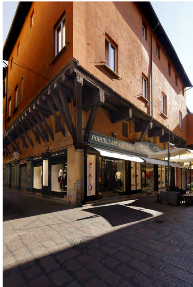
Fig. 1: Wooden sporti between Via Clavature and Via Drapperie.
