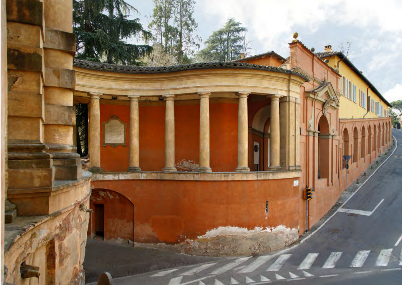
Fig. 49: Meloncello Arch, detail of the covered path to San Luca.
