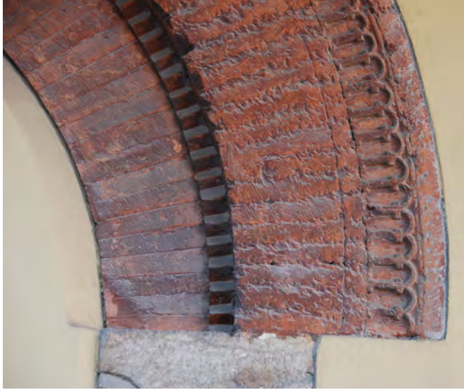
Fig. 12: Detail of the Romanesque archivolt under the portico of Case Tacconi Beccadelli, Via Santo Stefano 19.
