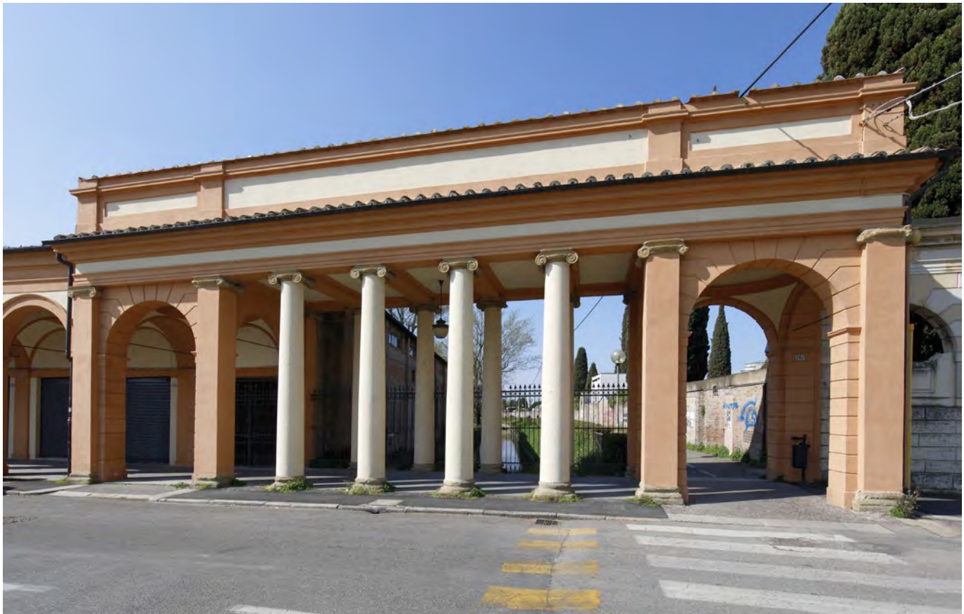
Fig. 56: Portico of the Certosa, porticoed bridge across the Reno Canal.
