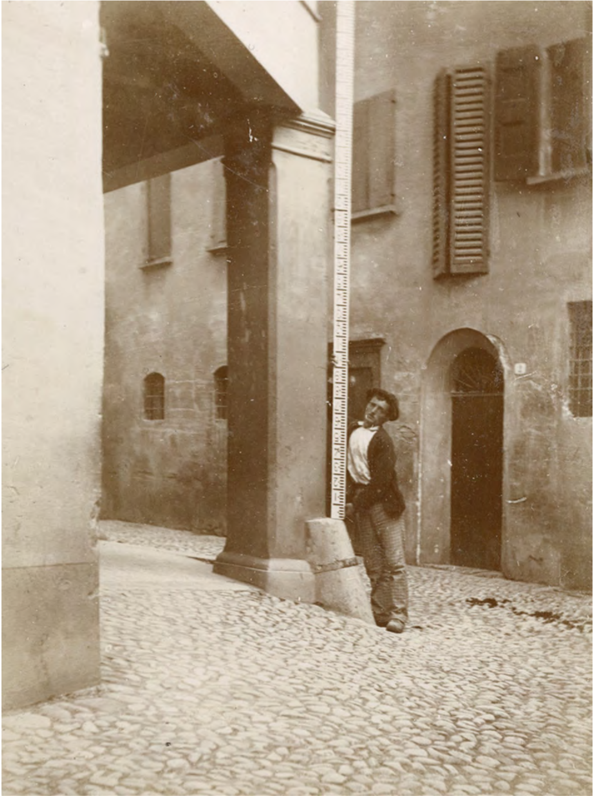
Fig. 63: Road leveling in Via San Bernardino (1896-97).
